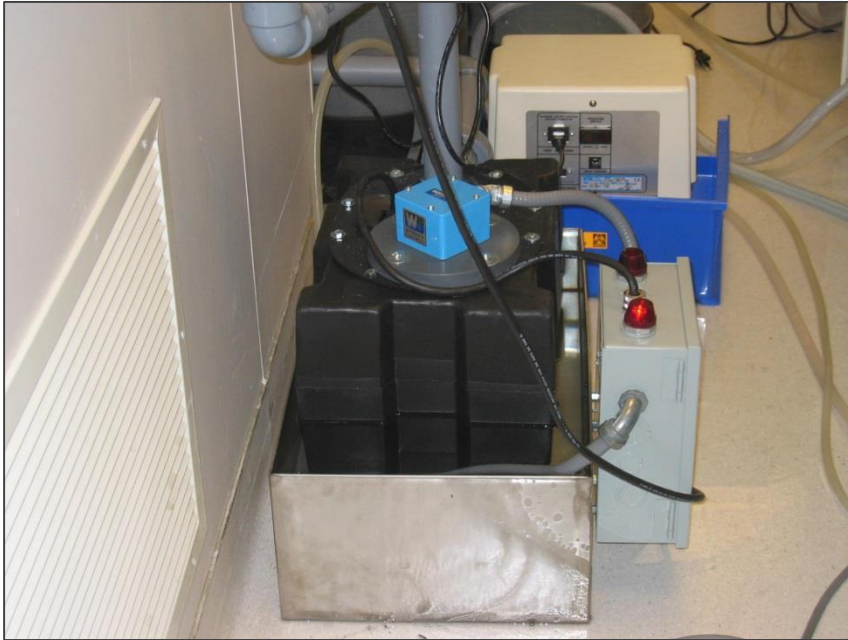
Treatment and pumping system for instrument waste
